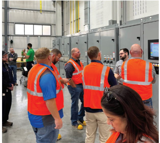
In the photo above, a long section of paralleling switchgear is tested at the Rehlko factory with generators in the next room.
